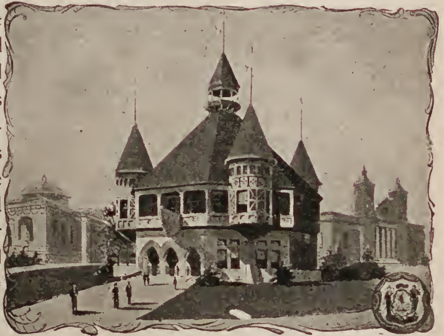
MAINE STATE BUILDING.
